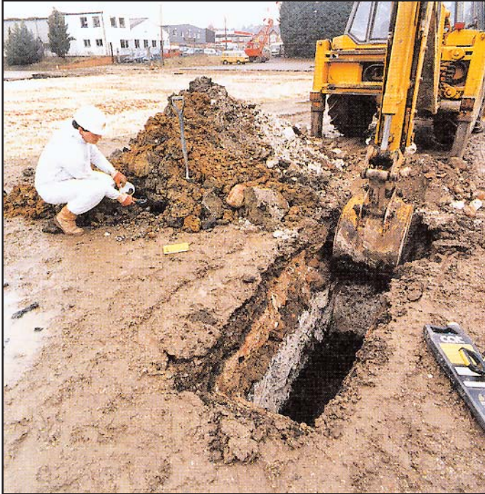
Trial pitting in potentially contaminated soil
