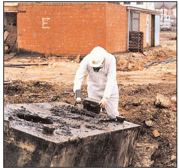
Monitoring of VOCs in buried storage tank
