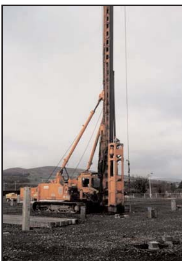
Pre-cast concrete piling rig
