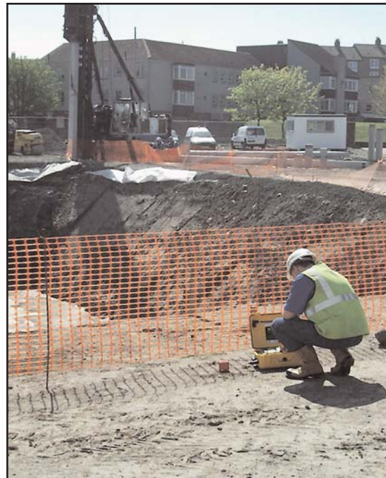
Setting up a logger during piling
