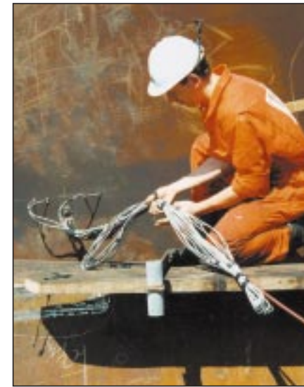
Pile Instrumentation Mounting
