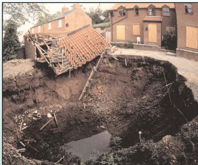
Above: Photo of subsidence due to gypsum dissolution. Ripon. N. Yorks 1997
