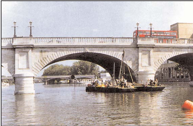
Investigation for proposed widening of road bridge
