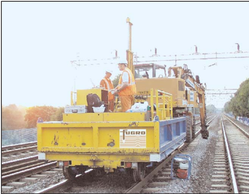
CPT Rail Rig - VAB Certified
