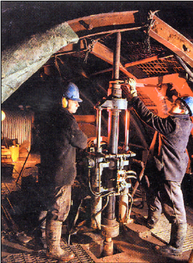
Conventional rotary core drilling of canal tunnel lining and surrounding ground
